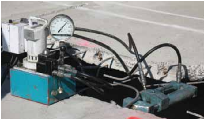
Fig. 10: Reseating an existing tendon anchorage. A slot for an external tendon is visible behind the pump
