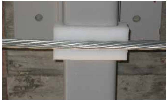
Fig. 8: Detailed view of HSS deviator, high-density polyethylene saddle, and galvanized strand
